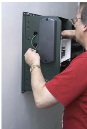
Figure 8 Placement of HUB.
